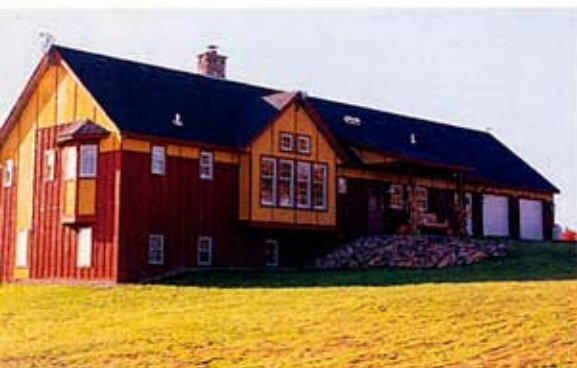
Board-and-batten siding stained red and yellow enlivens the exterior above. Dormers and secondary gable elements visually divide the roof's long ridge line.
